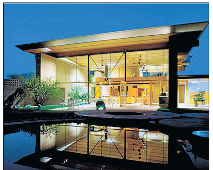
Green Broker offers high level results through many years of experience and a close understanding of the construction industry.
