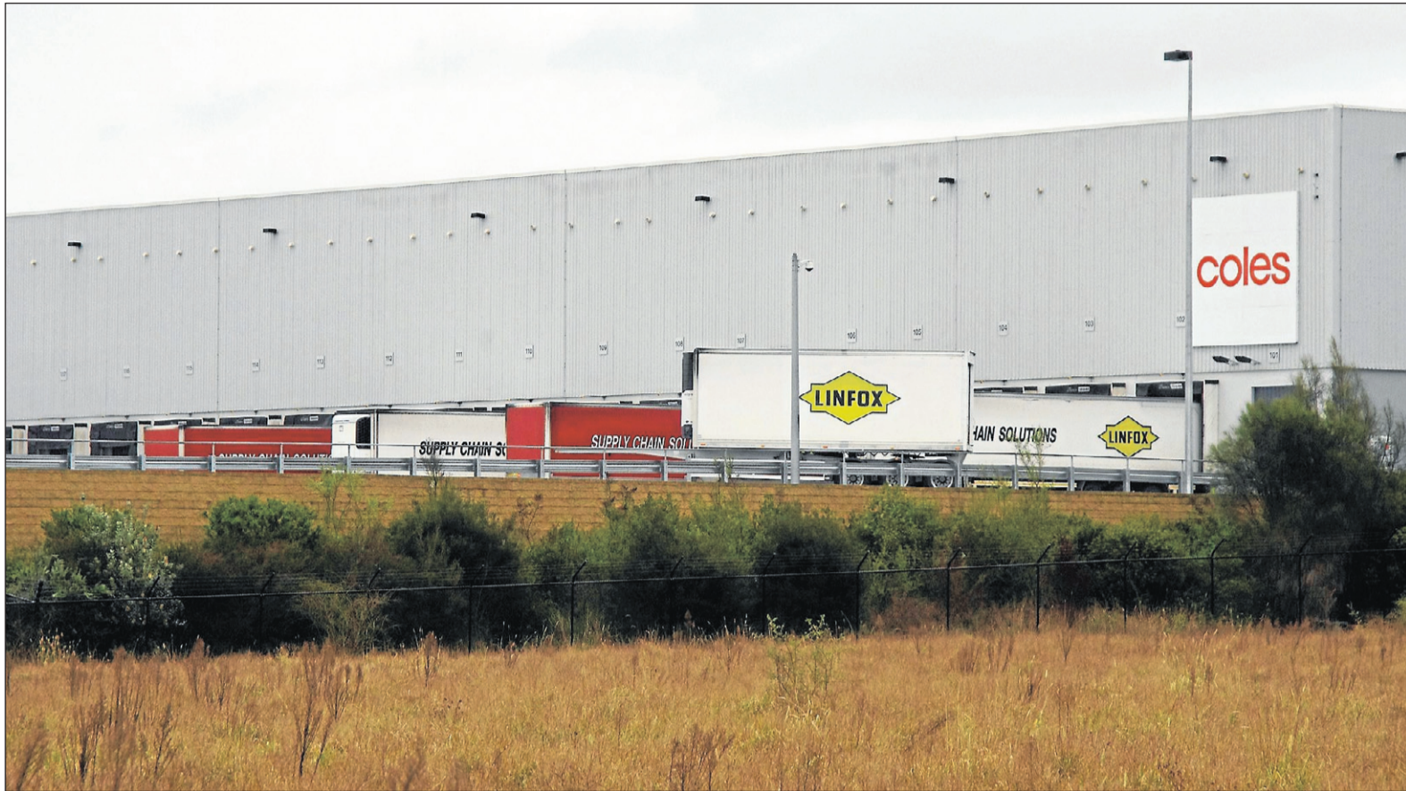
GOING NOWHERE: Work ground to a halt at the Coles Distribution Centre on Wednesday when staff say they were stood down by management following industrial actions in Melbourne. The company, however, says employees walked off the job in protest.
