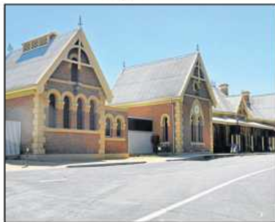
The former Young Railway Station is now Young's Visitor Information Centre
